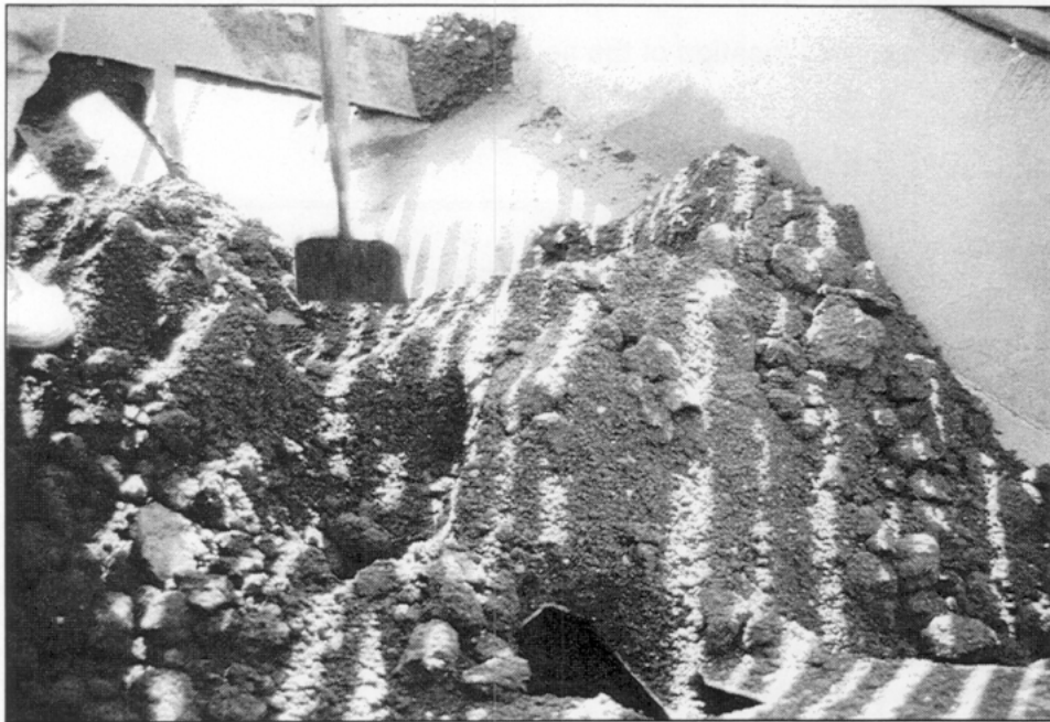
Figure 4. Working Inside Hopper to Breakup Clumps of Shingle Scrap
